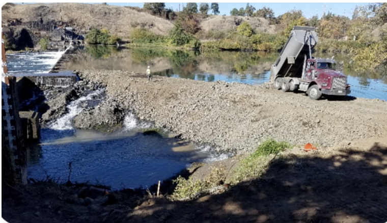
Construction of Unpermitted Cofferd Dam at Winchester Dam's South Abutment During Botched 2018 Repair. Photo courtesy of Oregon Water Resources Department
