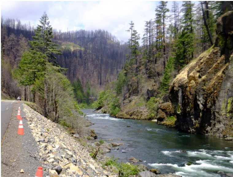
RipRap/Elevation Rock After the Archie Creek Fire: Photo by Lenny Volland
